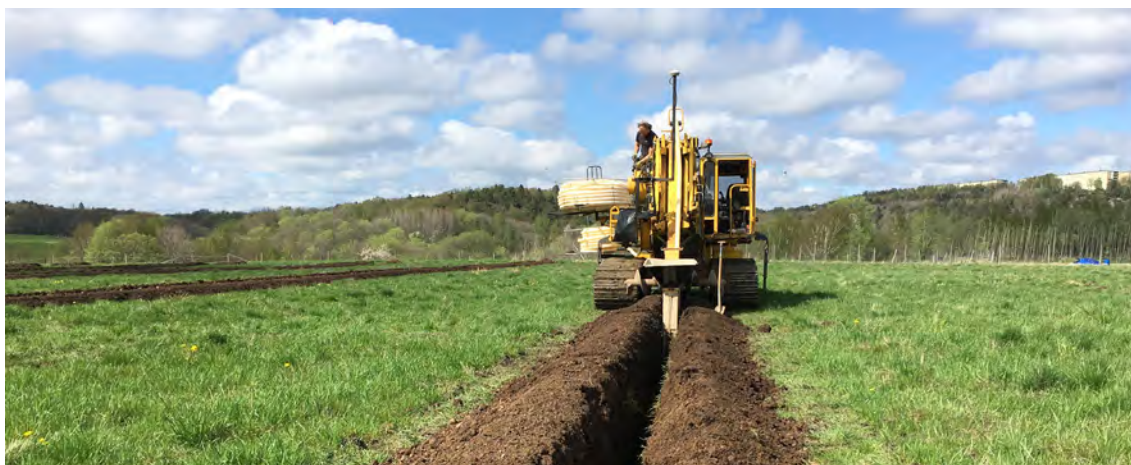
Figure 62 Installation of a drainage system at the test field for agroforestry at Naturbruksförvaltningen Angereds gård, Sweden. Photo by Mauricio Sagastuy.
