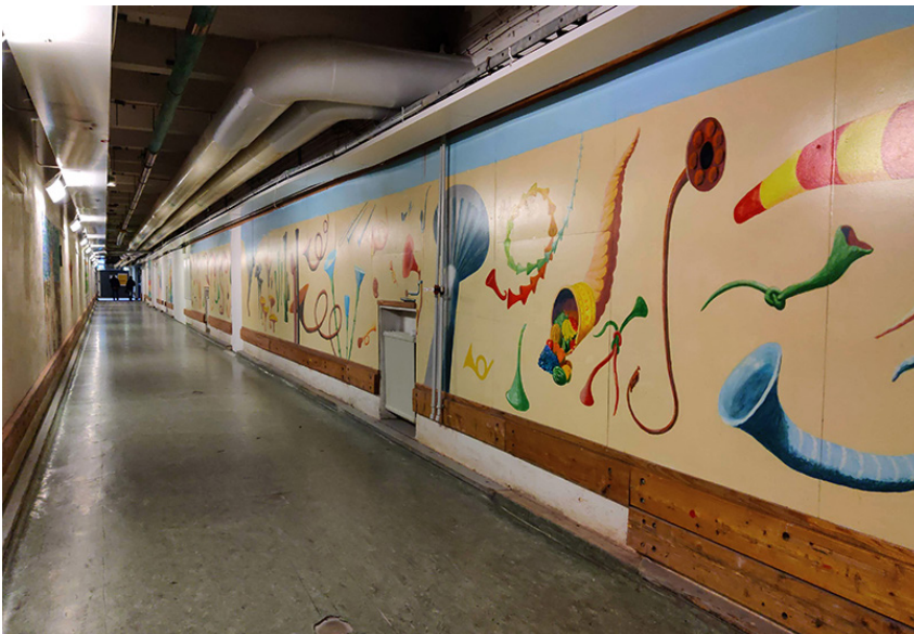
Culverts under Lillhagen. Photograph: Annika Engström 2021.
