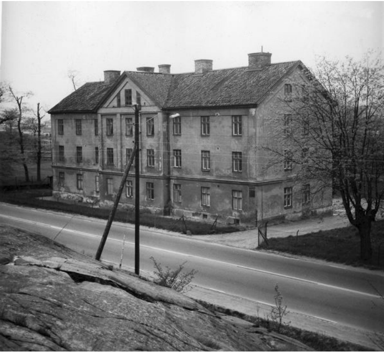
Gothenburg hospital in Gamlestan. Building demolished 1963.
