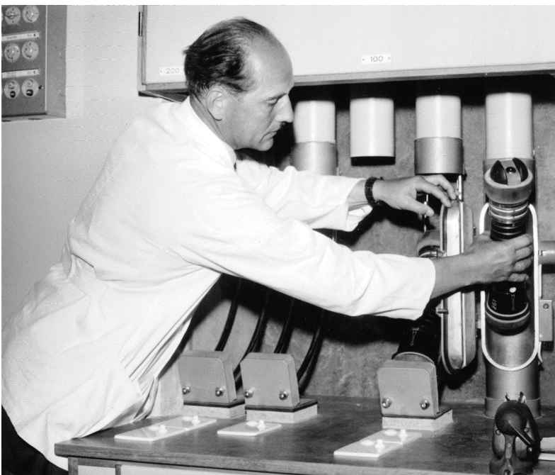
Vacuum pipe system at caretakers post, Sahlgrenska hospital 1959.
